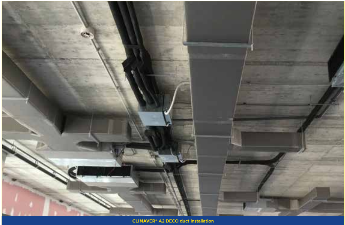
CLIMAVER® A2 DECO duct installation
