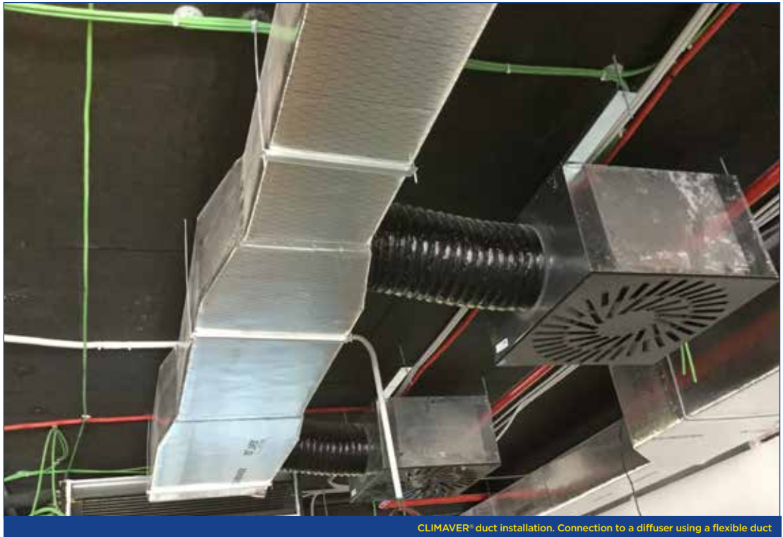
CLIMAVER® duct installation. Connection to a diffuser using a flexible duct
