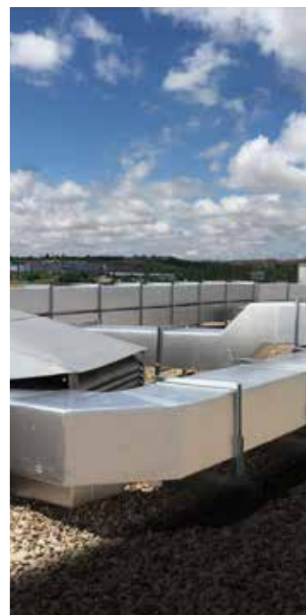
CLIMAVER® STAR duct installation
