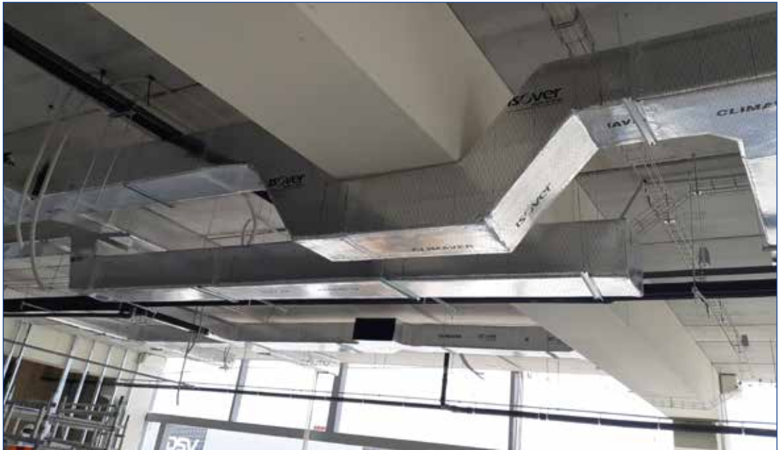
CLIMAVER® duct installation SDM Beampass
