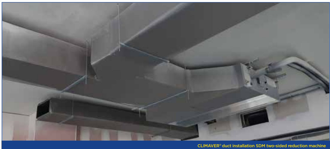
CLIMAVER® duct installation SDM two-sided reduction machine
