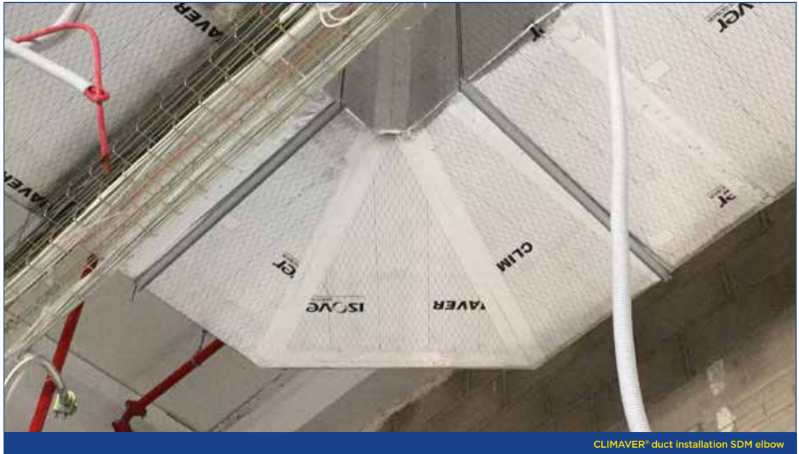
CLIMAVER® duct installation SDM elbow
